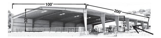
This agricultural building has several large openings in the building envelope. On the windward wall, there is a large 200-foot-wide by 25-foot-tall opening. On the two side walls, there are matching 100-foot-wide by 30-foot-tall openings. The leeward wall and roof have no openings.
